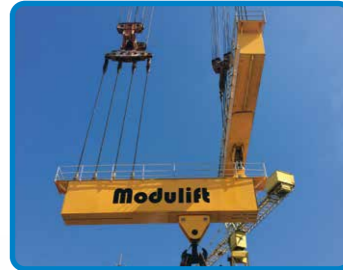
Lifting rig Harland & Wolff
